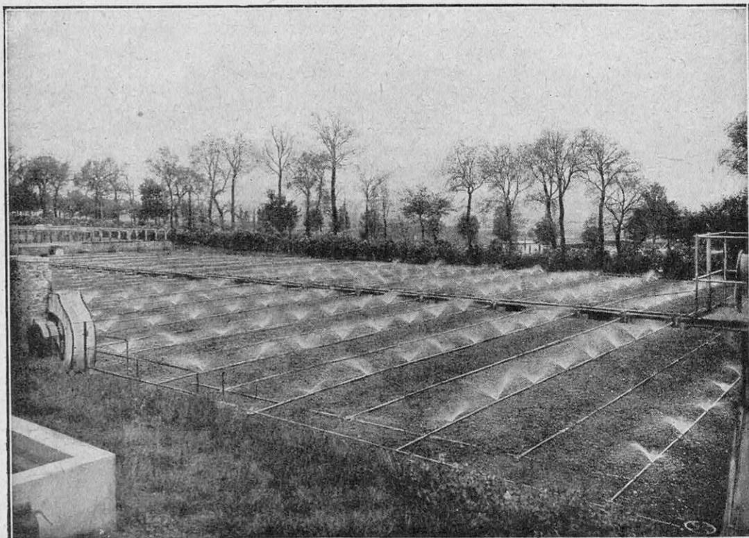
FIG. 2. — PULVÉRISATION DES EAUX D'ÉGOUTS SUR UN CHAMP. LES MICROBES AÉROBIES CONTENUS DANS CES EAUX ONT UNE ACTION FERTILISANTE (MONT-MESLY, SEINE)
